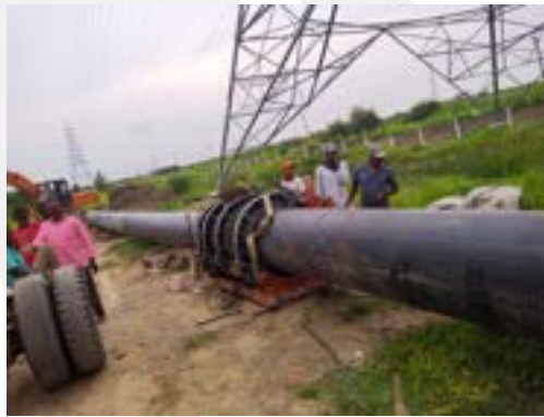
Heating process for bid forming
